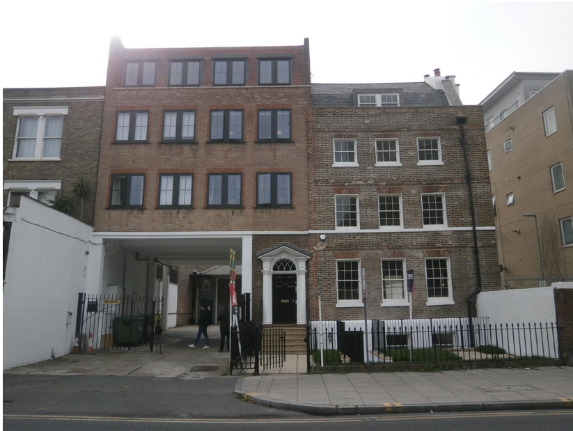
Front of Grade ii 160 Dalston Lane
