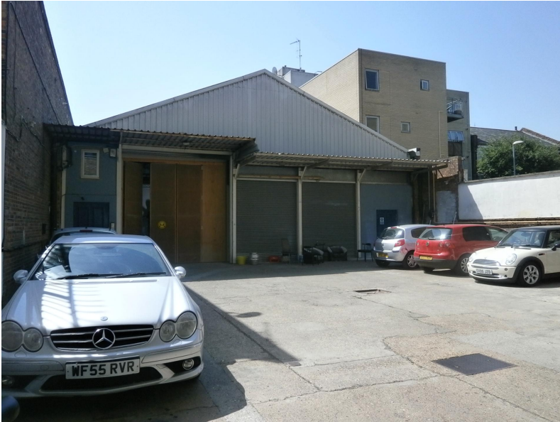
Existing warehouse building
